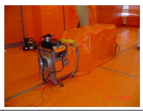
P1 Negative air unit set-up to be DOP/PAO Tested using the mixing chamber method.
